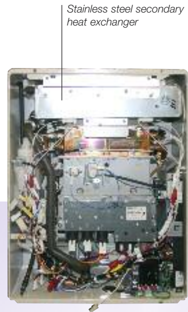
FASTflo – PLUS Condensing model Internal view
